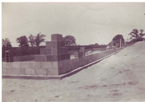
Joe Gurka's motel in Maryland, at about the stage of construction it was in when he learned that the road was soon to be moved.
