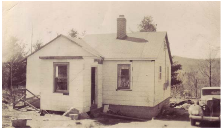
Martin Gurka's house on Tarringford West St., Burrville, in early development, around 1940.
