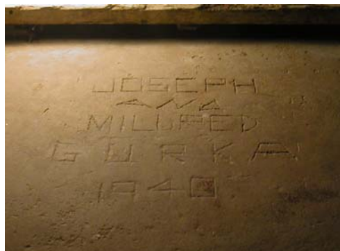
Dad inscribed this in the cement of the cellar floor, at the foot of the steps.
